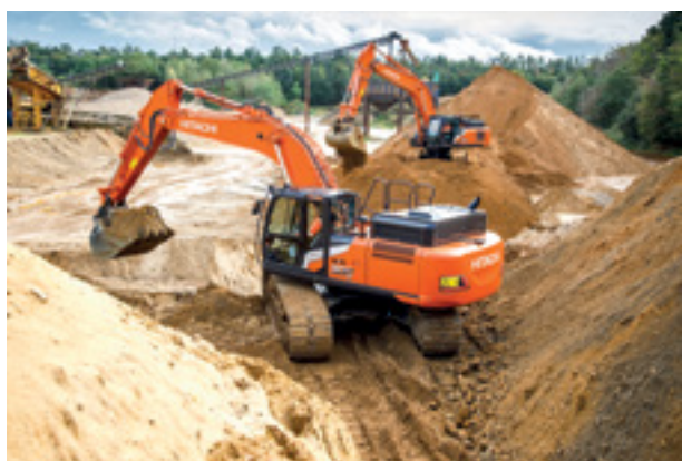
Zaxis medium excavators
